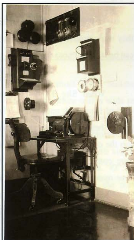
Photo 9: A view of the teletype desk area. Compared to Photo 6 this must have been after the telephone was installed.
