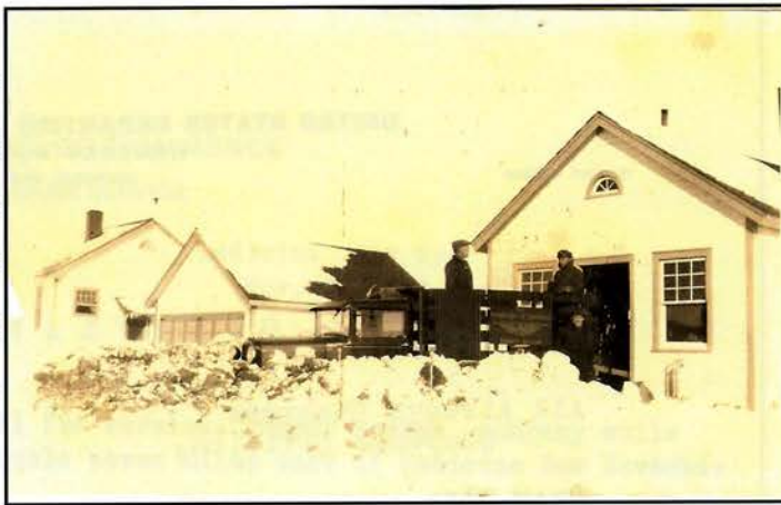
Photo 18: This shot of the power house was taken before the elevation numbers were painted on .
