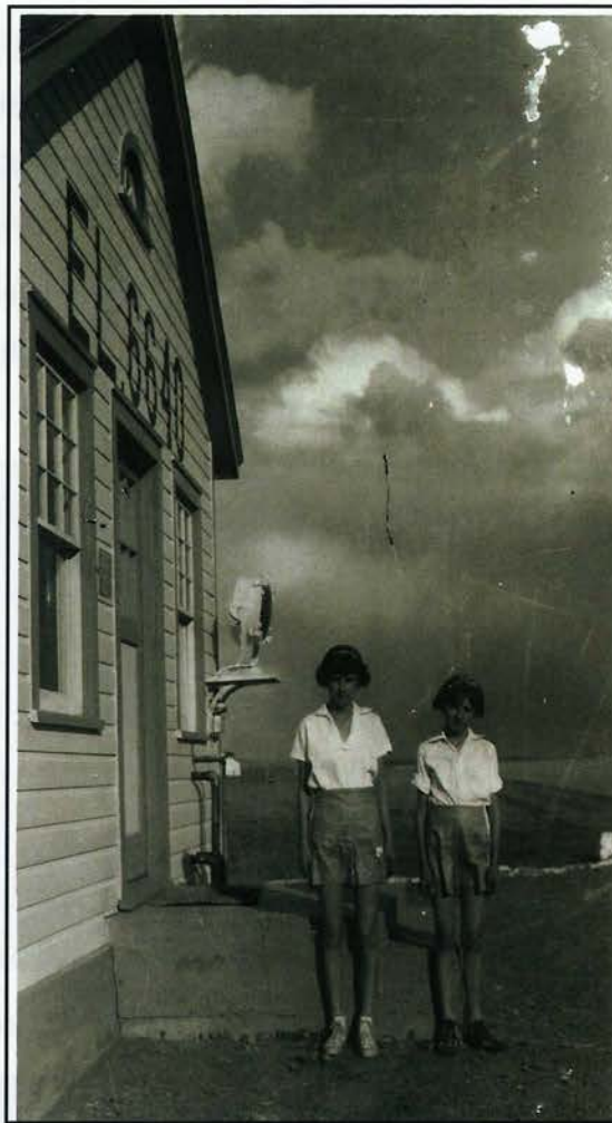
Photo 30: Betty and Evelyn outside the power house; c.a. 1934
