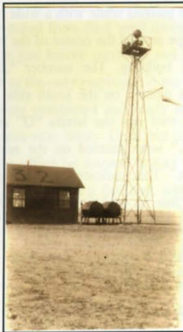
Photo 3: Office building and tower at Site 32, picture #1; c.a. 1930.
