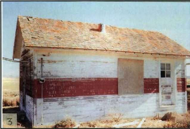
Photo 33: Office building looking SW (Steve Wolff-
