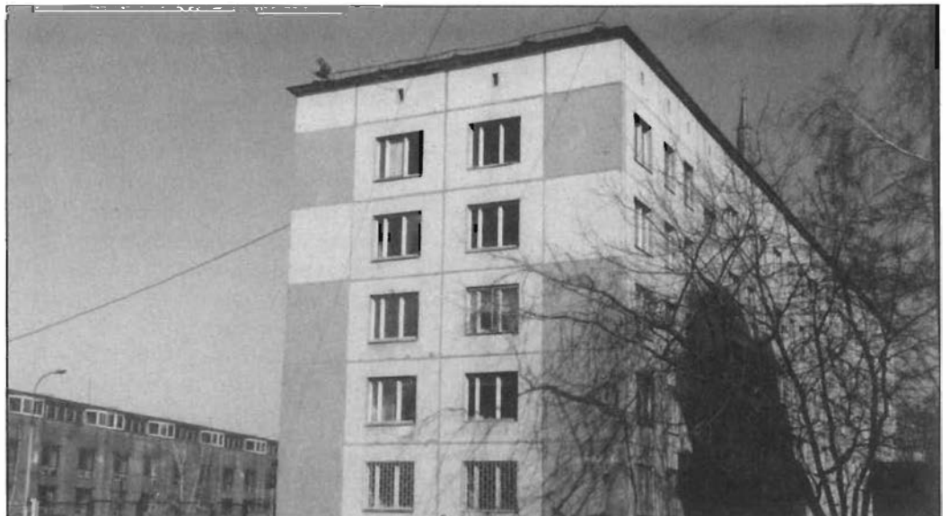
The building that the FAA is in. New American Embassy on the left.
