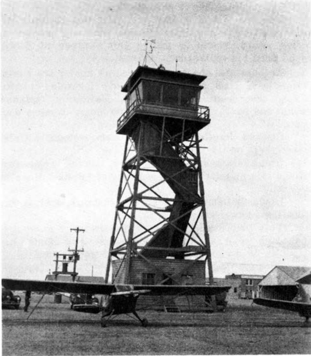
Old Merrill tower, landmark for the past 20 years, retired from service.
