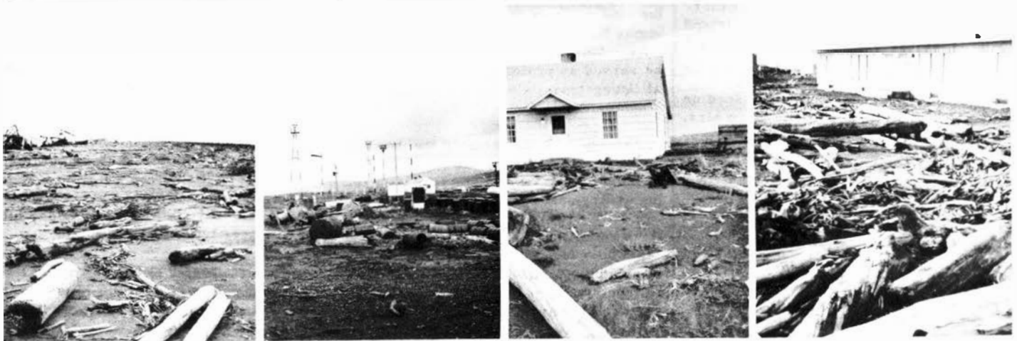
FLOOD DAMAGE AT UNALAKLEET
