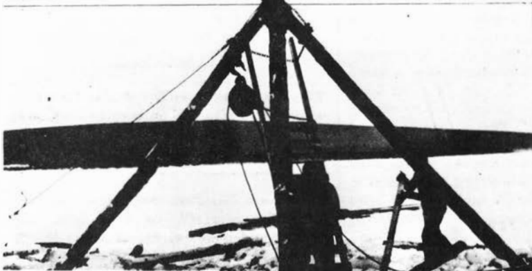
BUSH ENGINEERING--THE ELEVATOR IS READY
