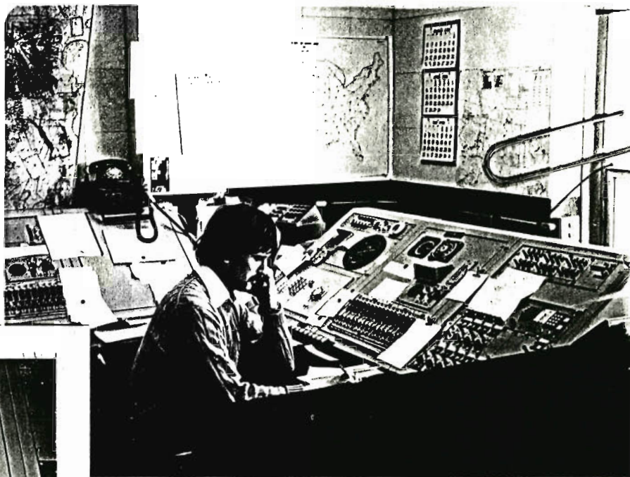
Some of the new FSS Equipment
