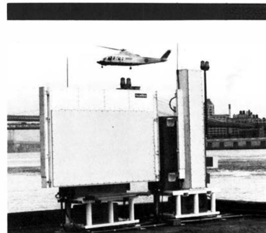
*An FAA helicopter makes a demonstration flight to the microwave landing system-equipped Wall St. Heliport in New York City. Only a heliport has the elevation and azimuth antennas collocated. The agency presently has 170-plus MLSs on order, including systems for three heliports.*
