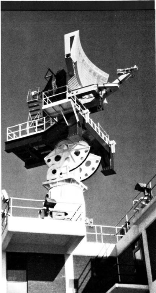
*The first production system of the Westinghouse ASR-9 Airport Surveillance Radar is being tested by the company near Baltimore-Washington Airport. The first of 132 FAA and DOD systems will go to Huntsville, Ala., for FAA testing in July 1986. The new radar will detect six weather levels, low-flying aircraft and aircraft on tangential courses.*
