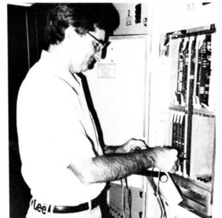
Maintenance technician Spiro Tsongalis tests circuitry in the equipment room of the Bridgeport FSS.
