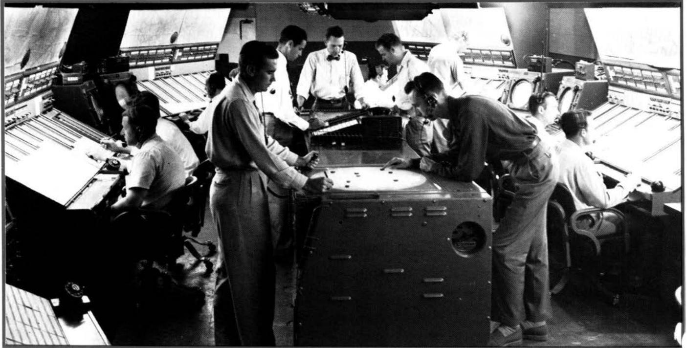
The Washington ARTCC in 1955 used surplus Navy VG (video generator) "battleship" radars with plastic shrimp boats. Along the walls were plan position indicators, radars used to service certain airspace sectors.
