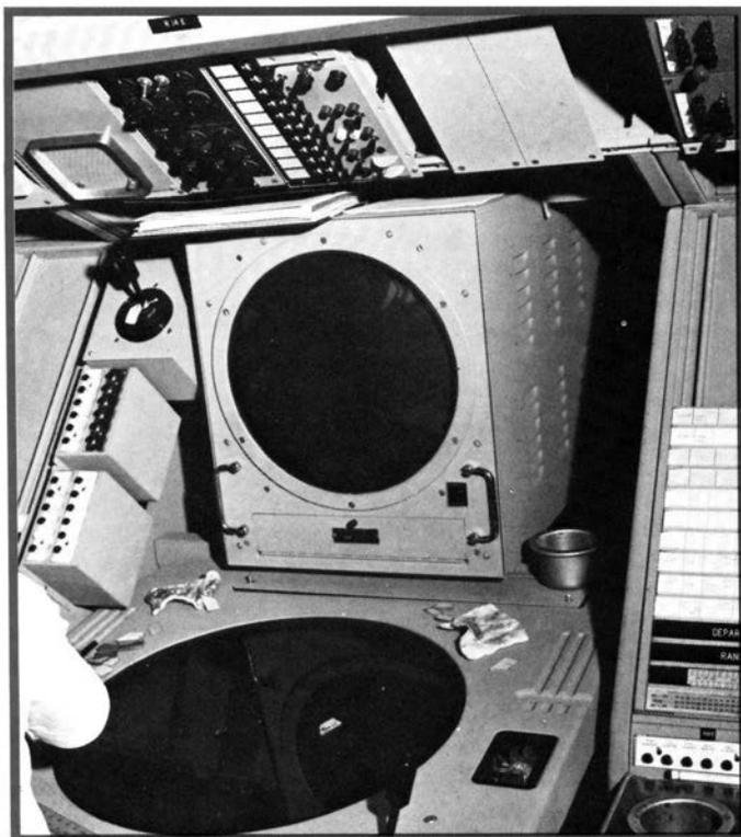
*In 1963, air route centers had radar bright detection equipment (RBDE-5). In some, the supplemental vertical display was just for backup; in others for split sectors or ranges or for separating approaches and departures. Controllers used plastic shrimp boats, grease pencils and cleaning pads all day long.*
