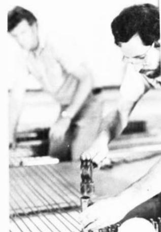
*Dick Forsythe, engineering technician, installs a brake wire system which stops the sled on which the seat is mounted. The sled is pushed by a 5,500-pound weight.*
