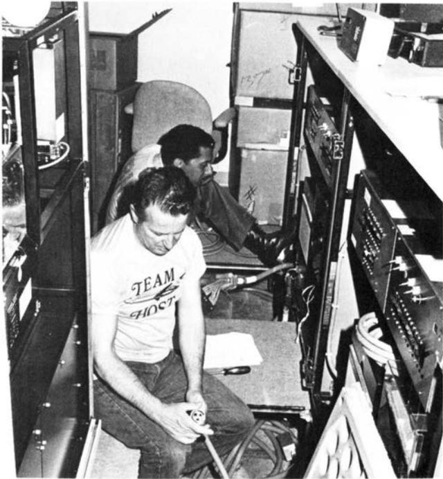
*IBM technicians with their backs to the host computer attach cables to the 9020 interfacing switch.*
