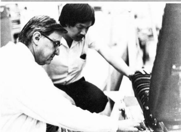
*Dick Chandler (left) confers with Dave Gee of Beech Aircraft about one of their donated seats prior to testing for energy absorption, the adequacy of seat restraints, the reliability of attachments and hardware and its overall construction.*
