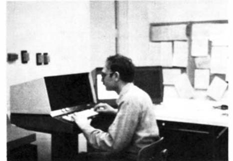
The central control monitoring system computer is used by utility systems technician Anthony Vangeli to check out the TRACON's environmental systems.
