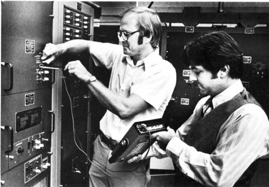
Student Larry Himli plugs into the VORTAC's power supply as instructor Don Torchio demonstrates the use of a multimeter in checking the equipment's internal voltages.
