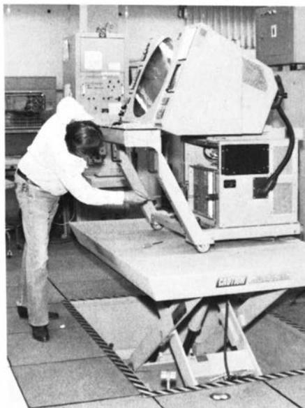
Glever Murray, computer display channel technician, has a 660-pound display on the PVD lift for hard-to-get-at adjustments.
