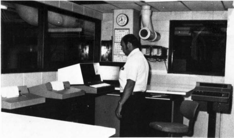
Harvey Burr, assistant chief of the Chicago ARTCC's environmental unit, checks status of the air conditioning system throughout the building with a computerized remote maintenance monitoring system.
