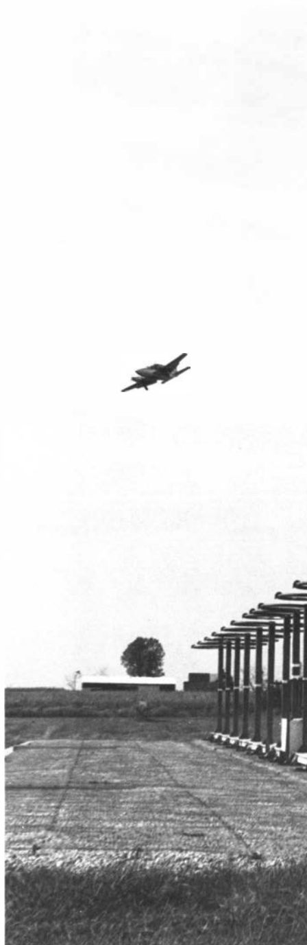
A V-ring localizer antenna for the Burlington, Iowa, instrument landing system sits at the approaches to Runway 36.
