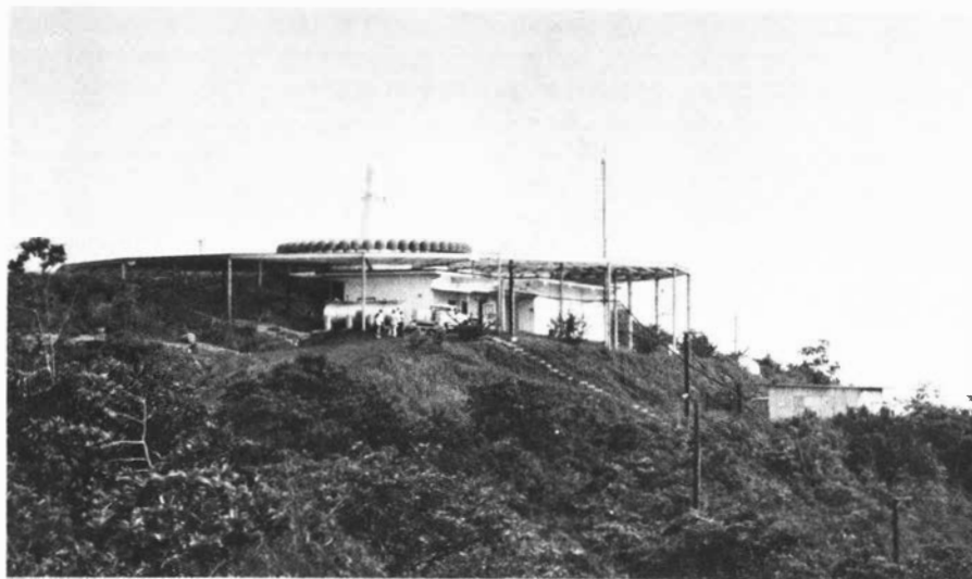
A doppler VORTAC on Taboga Isle, Panama. All are being converted to solid-state.
