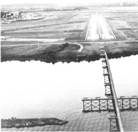
Improvements to approach lighting systems will make them switchable when visibility permits to effect energy conservation.
