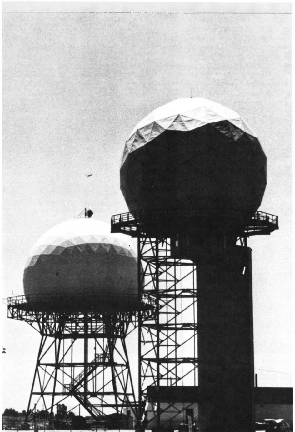
The ARSR-3 long-range radar (right) dwarfs its predecessor in Mcook, Ill.
