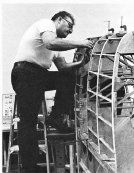
Museum technician John Cusack restores the wing of a Northrup 1NM Flying Wing, carefully regluing joints and replacing dryrot with faired in pieces of wood.
