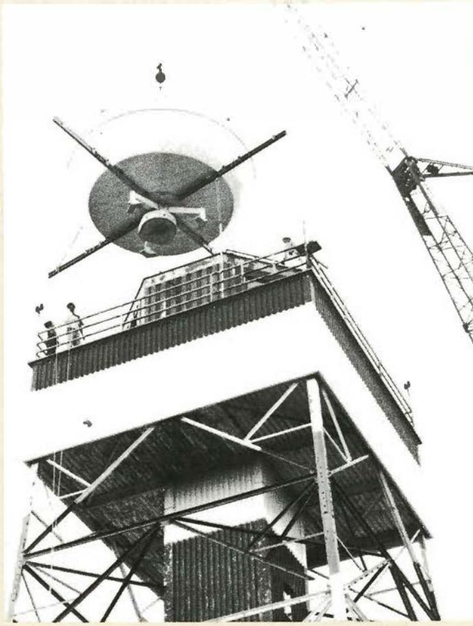
**NEW AIRPORT RADAR**—Work crews install a new Airport Surface Detection Equipment (ASDE-3) radar at NAFEC/Atlantic City Airport where it's undergoing test and evaluation. The Cardion surveillance radar is expected to increase safety and reduce delays at more than 30 major airports.
