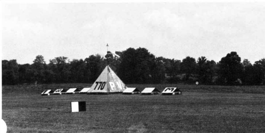
The identifier pyramid, bearing the airport's initials and altitude, is topped with a windsock and floodlights. The markers indicate runway headings of 18 and 36, with the farthest left one bearing a red mark for a displaced threshold.
