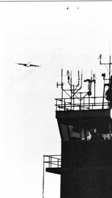
The heart of air traffic control: communications antennas sprout from the roof of a tower like weeds after a spring rain.
