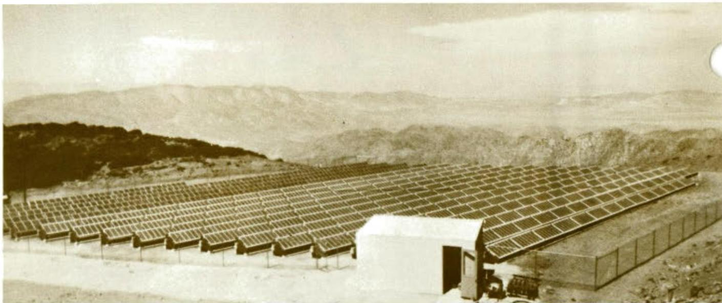
The field of photovoltaic cells that helps power the Mt. Laguna Air Force Station and Los Angeles Center radar occupies half an acre. The power system's output is 60 kilowatts.
