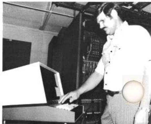
Don White, Wichita, Kan., technician-in-depth, checks a readout on a portable terminal of information from a remote monitoring system under test at a radar site near Hutchinson, Kan. The purpose is to save unnecessary trips to the site to check the functioning of its equipment.
