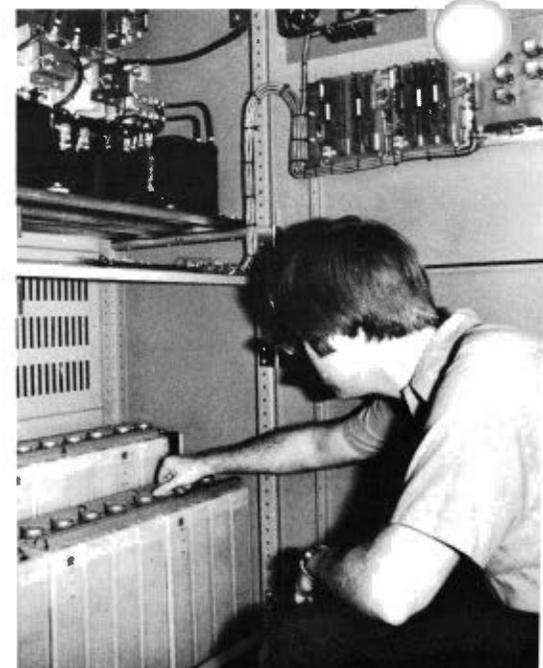
A new battery emergency power system under test at the Hutchinson, Kan., RCAG site, expected to replace petroleum generators, is checked by engineer Randy Downing.
