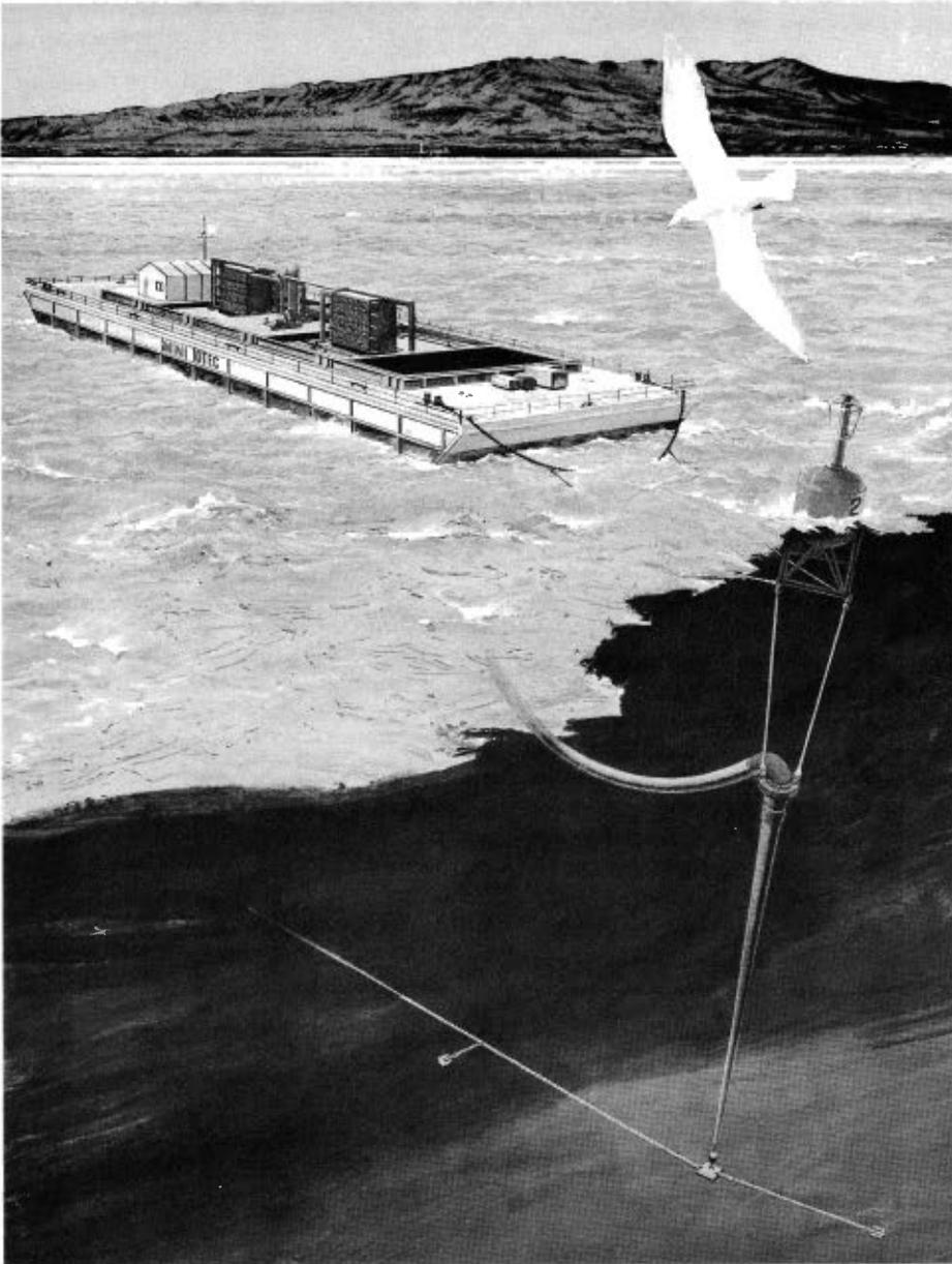
**A** mile and a half off shore from Ke-ahole Airport, which serves Kona, Hawaii, is an anchored Navy barge producing electricity without using fuels. It's the world's first Ocean Thermal Energy Conversion (OTEC) plant.
