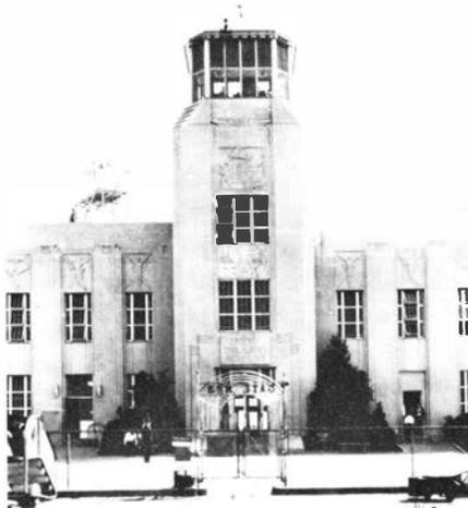
*Right: The first air traffic control tower in the U.S. was this one at Cleveland, Ohio, in 1930. The device on top of the greenhouse cab is a wind "tee."*
