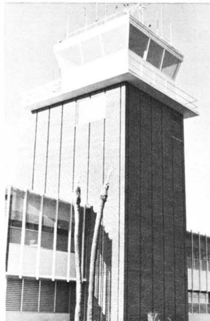
*The Tallahassee, Fla., tower (below left) is not a modern version of terminal combination, but it is combined with a flight service station and the Weather Bureau. Note the four-sided cab, notorious for its reflections.*
