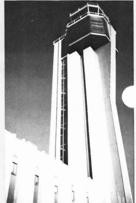
El Monte, Calif., sports a 1972 functional-shaft tower, but there wasn't room to put the stairway inside the structure (below left).
