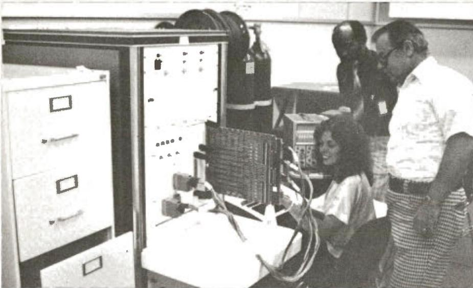
**RADAR BACK-UP IN PLACE**—Electronics technician Bob Hayes (right) shows technician trainee Sue Leech the operation of the Direct Access Radar Channel (DARC) printed-circuit-board tester recently installed at the Minneapolis ARTCC, while John Smith of Raytheon observes. A replacement for broadband radar, DARC will be undergoing shakedown tests at the Salt Lake City, Minneapolis and Chicago en route centers.
