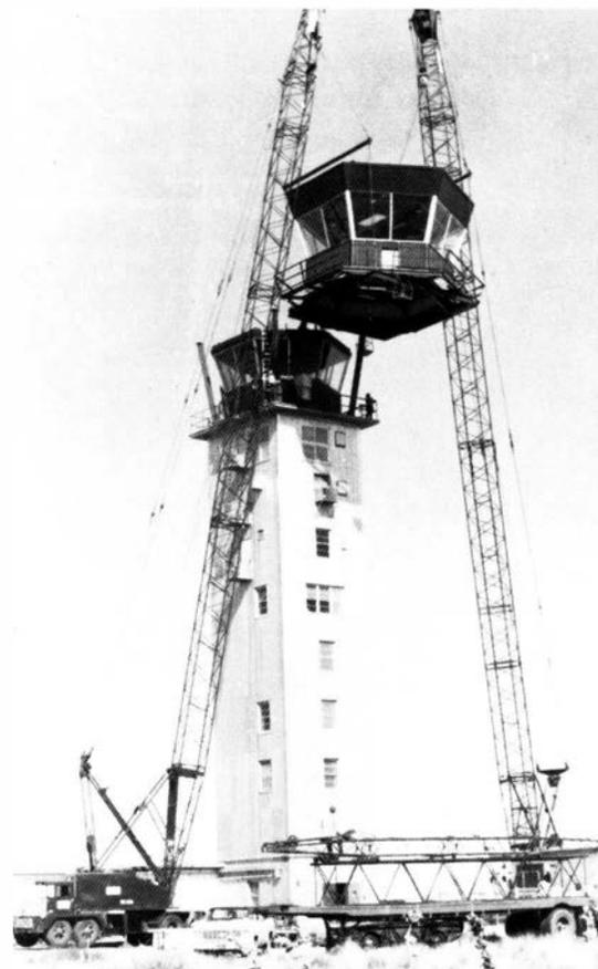
*The Albuquerque, N.M., tower got a crown upon its crown during a modernization designed to increase its height and space for more modern equipment. The old cab is now used for a training facility.*
