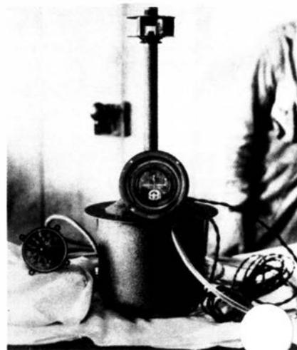
*The shaft of the earth-inductor compass passed through the top of the fuselage to catch the wind; the tub holds a rotating armature; the dial at left is for setting a heading; the other dial is a left-right indicator.*
