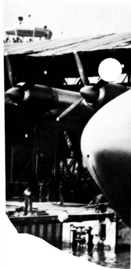
*Getting ready for the first flight of the HK-1. Technicians board the flying boat through the forward hatch.*
