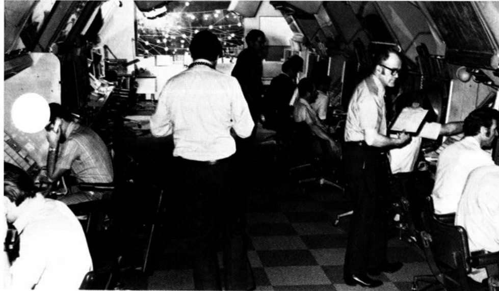
A recent view of the center. Radar scopes are in vertical positions, since electronic data tags—not shrimp boats—were used by controllers since 1963.
