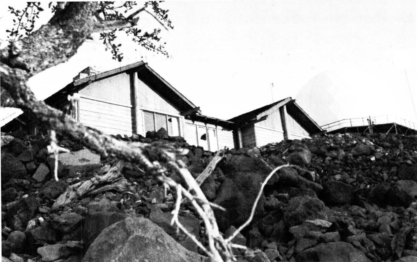
Home and the radome at Brushy Mountain.
