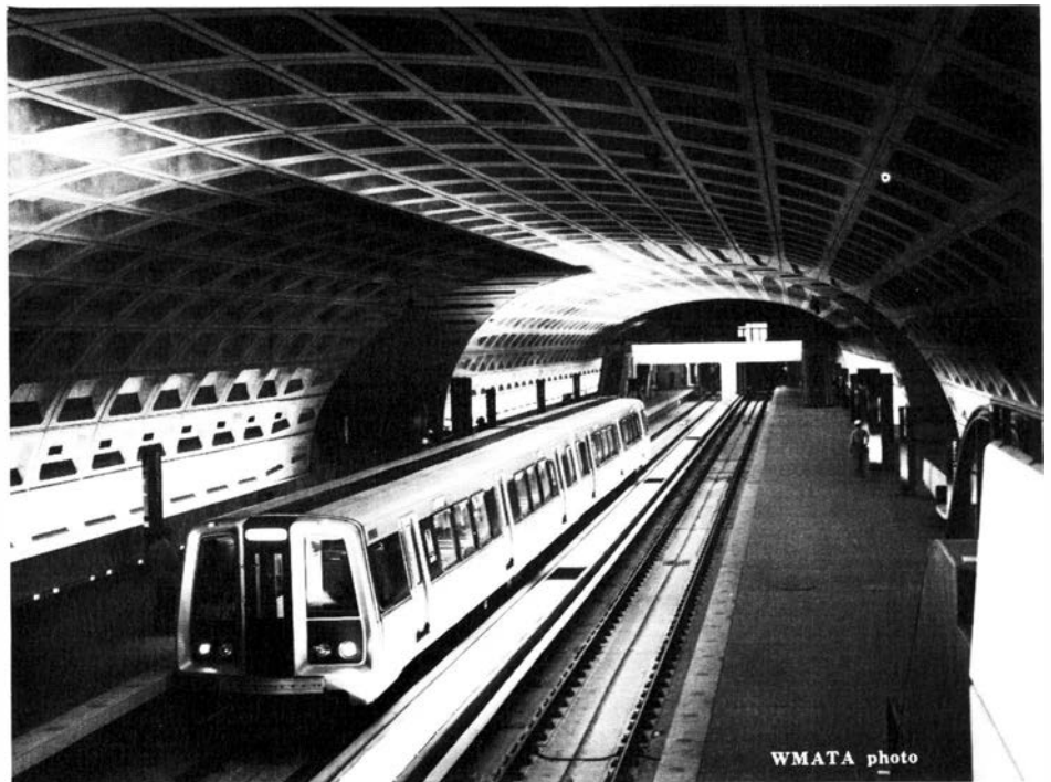
The Metro Center station at 12th and G Sts., NW, in downtown Washington is on the 4.6-mile leg which opens this month. Arched Metro station ceilings have no supporting pillars restricting the view of security attendants and closed-circuit TV cameras. The trains run on cushioned tracks and are so quiet that lights along the platform flash 20 seconds before a train arrives to warn waiting passengers.
