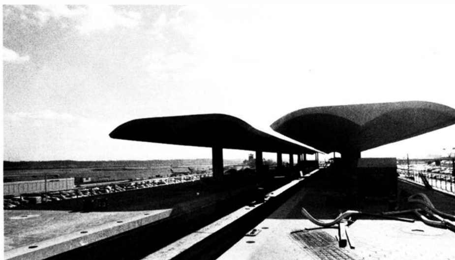
Metro's above-ground stations, including this one at National Airport, are marked by a graceful gull-wing canopy for passenger shelter. It's windy up there; however, the platform benches will be protected by glass screens.
