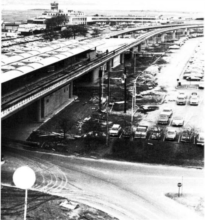
The Washington, D.C., Metro rises in Virginia to be an elevated structure and runs to National Airport between Rosslyn and Alexandria. The main airport terminal is in the rear, right of center photo, and the airport access road passes under the Metro station in the foreground.
