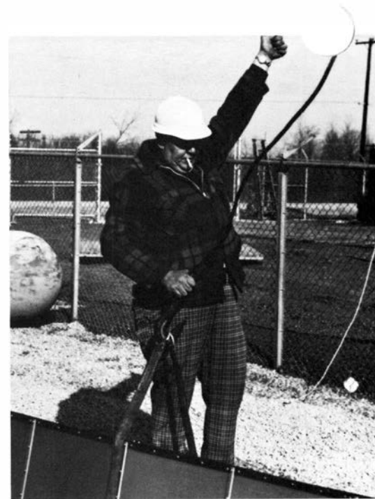
Take 'er away, signals supervisory electronics technician John Kubiel after securing a cable to the beacon antenna.
