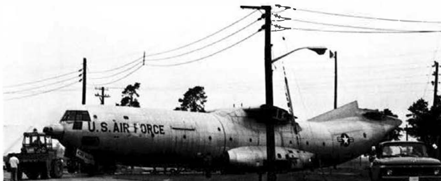
Moving day at NAFEC: The fuselage of a surplus C-133 Air Force cargo plane was moved from one part of the center to another for use in testing burning cabin materials because of its similarity to a wide-body jet.
