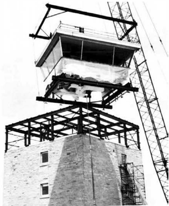
The 25-ton tower cab at the University of Illinois-Willard Airport was removed to make way for a one-story addition, then replaced and operated while the floor below was being completed.
