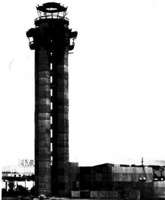
Atlanta International Airport's new tower under construction is getting the installation of enhanced ARTS III.
