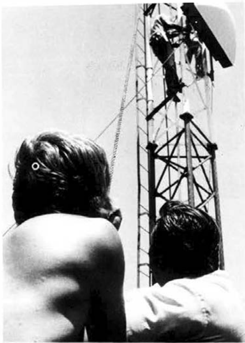
Airway Facilities technicians raise a portion of a glide-slope antenna at O'Hare International Airport. Solid-state glide slopes were among the new instrument landing system components installed at airports in the Great Lakes Region this past summer.
