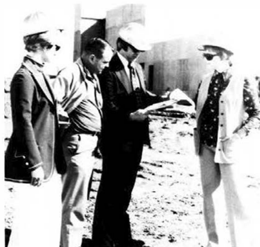
At the construction site of the new Atlanta International Airport Tower last summer, resident engineer Wade Kemper (second from left) briefed contracting officer Steve Wright (center) and contract assistants Susanne Edge (left) and Fran Babb, hardhatted for the occasion.
