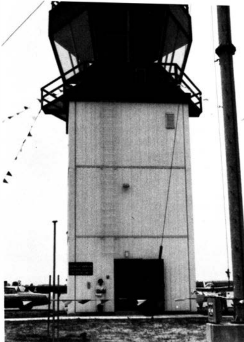
The last of five Central Region low-activity turnkey towers was commissioned in Cape Girardeau, Mo. Inspecting and monitoring all five, which were under concurrent construction, were David Henderson and John Gronberg.
