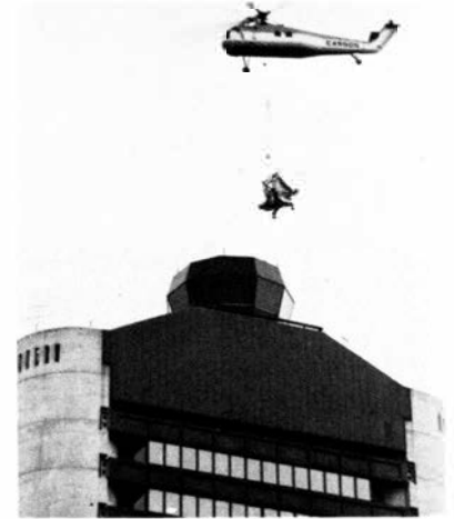
It took less than five minutes to transfer the one-ton radar antenna by helicopter from the old nine-story tower to the new 22-story control tower commissioned last month at Logan International Airport.
