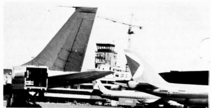
Framed in the hubbub at the Seattle-Tacoma International Airport, the new Sea-Tac Tower rises around the old one, the new cab perched two stories above the operating cab.
