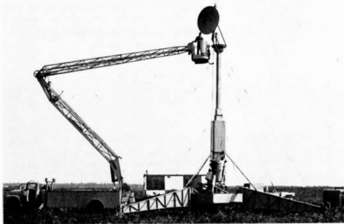
Perry Yon rides the bucket, Oscar Adams works behind the radar dish and Frank Rosati is on the base of one of the three radar beacon antennas being installed as part of a ground-based data-collection system for pattern measurements.
