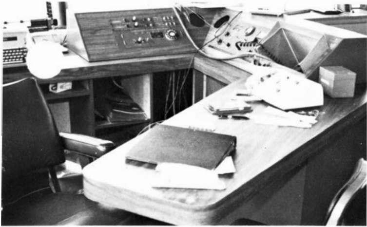
The nearly completed assistant chief's desk combines runway and control position visibility with monitor panels.
