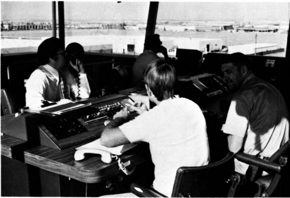
Controllers work their positions at the new homebuilt T-shaped console at the Santa Ana, Calif., Airport Tower. The old, high-angle turrets next to the cab windows obstructed the view and limited equipment servicing access.
