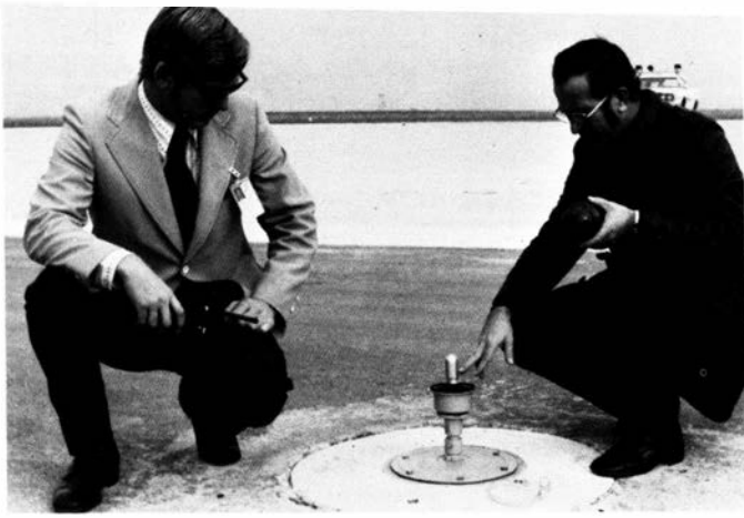
Inspector Staley (right) removes the globe to demonstrate the proper bulb alignment in a non-glare runway light to airport operations supervisor Ron Bowling.
