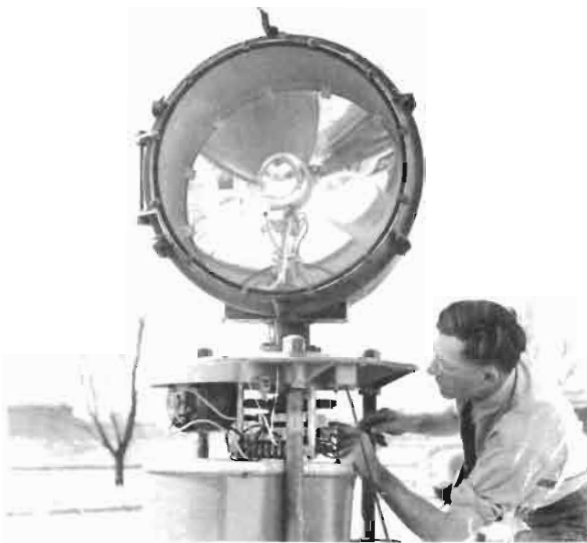
Cy Martin adjusts wiring in a 24-inch airway beacon.
