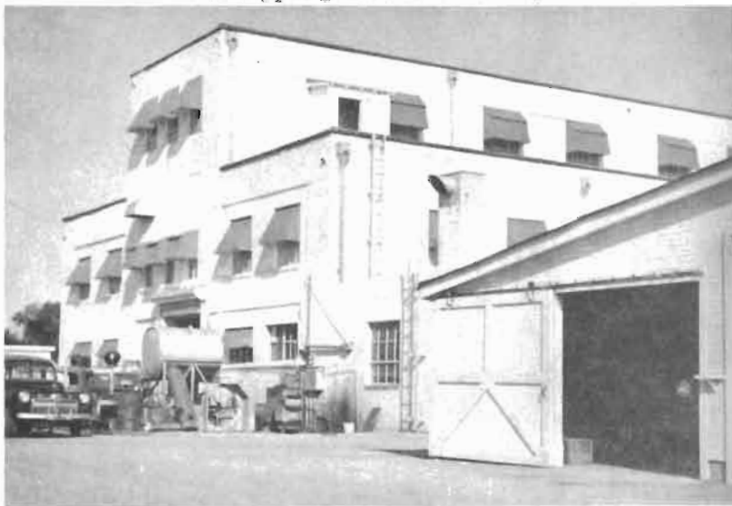
SOUTH END, BUILDING 2 (1948) Soon to be office spaces.
