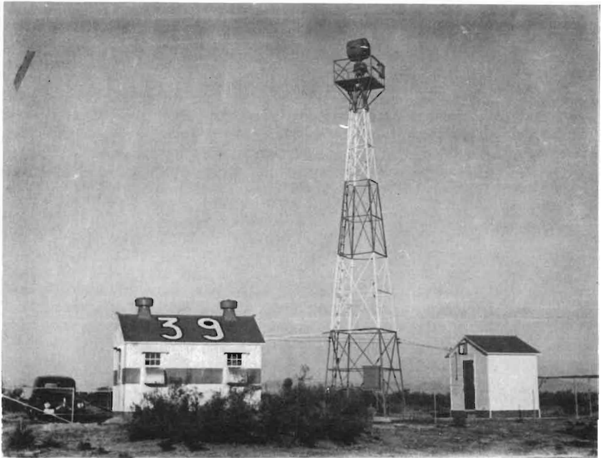
Beacon located at Harrington Ranch Field between El Paso and Columbus, N. M., on Los Angeles-El Paso Airway. Fan marker is also installed here.
