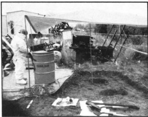
Bethel 1992, PCB spill; old electrical component put out in storage; less than 2 gallons of oil leak, 10 yards of soil removed
