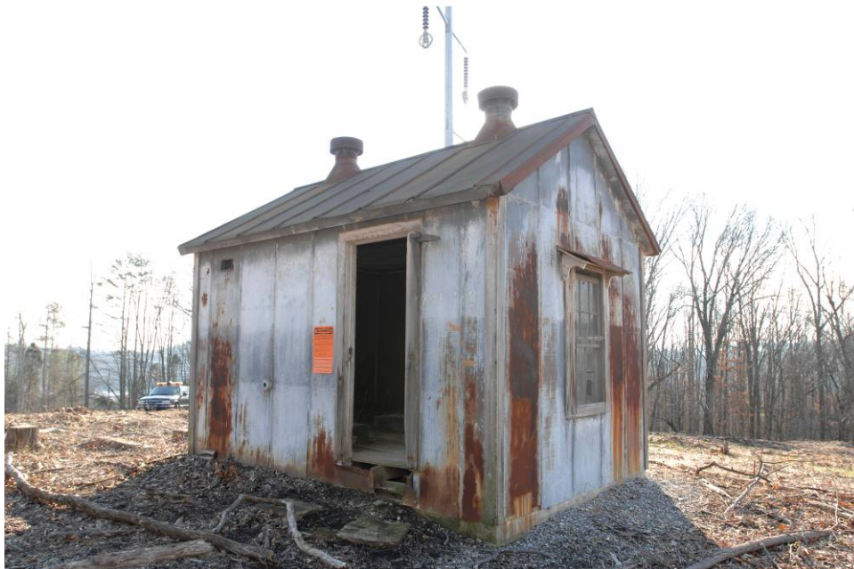
Fig. 1. Building 0969 on the Oak Ridge Reservation.
