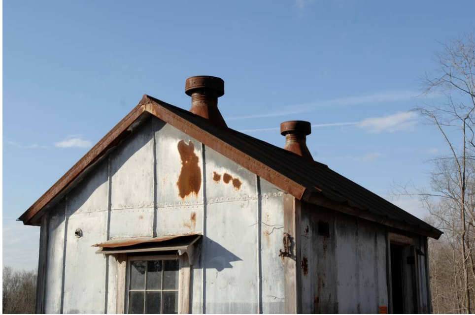
Fig. 5. The roof, vents, and siding, are rusted but not leaky.
