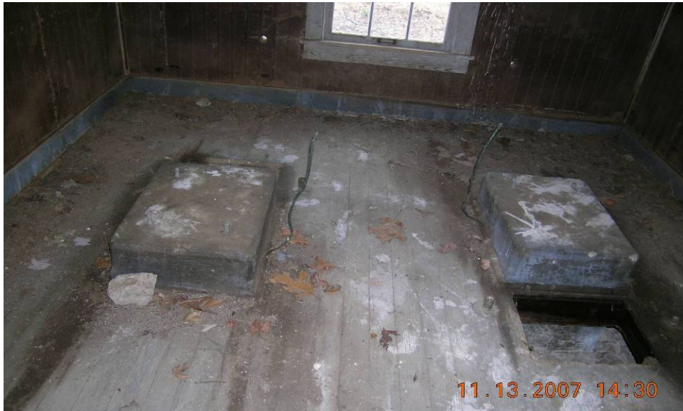
Fig. 4. The wood floor and the piers that supported the power generator.
