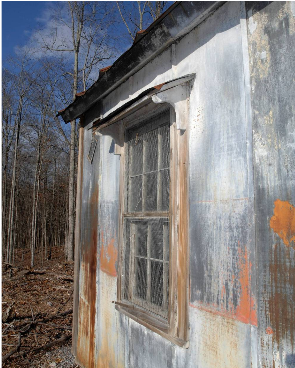
Fig. 2. The windows are protected by hoods.
