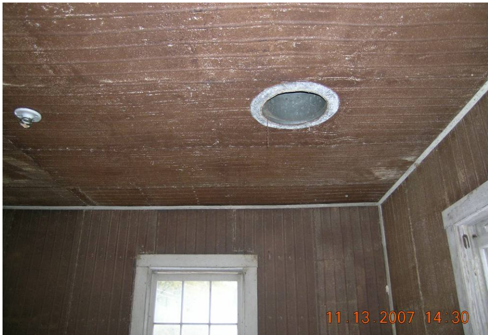
Fig. 6. Interior view: ceiling and walls.
